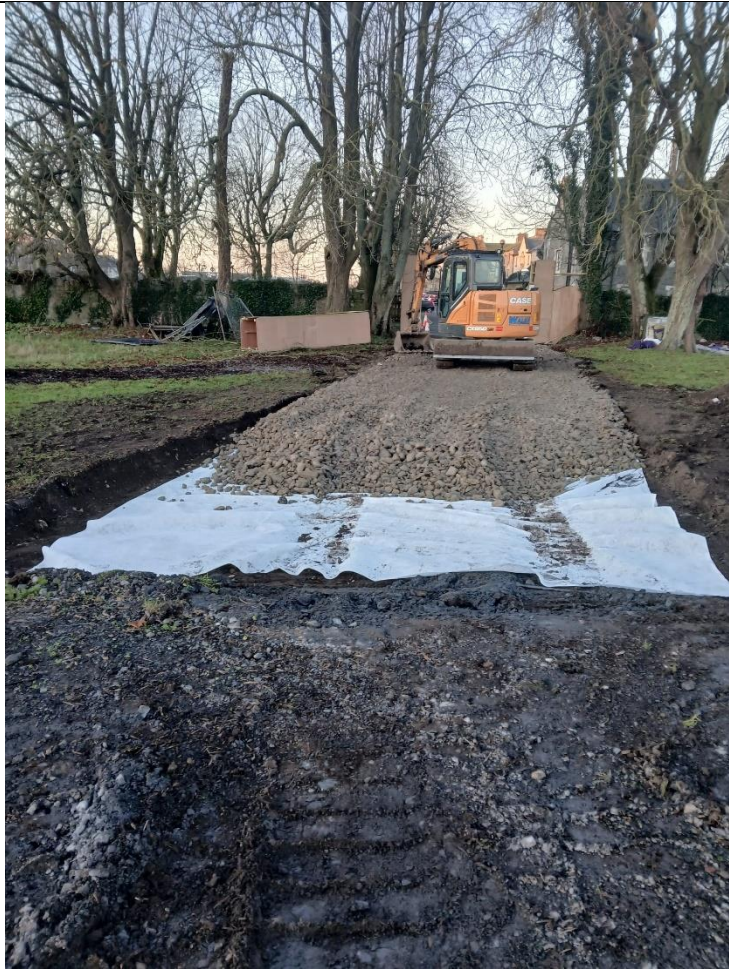
Date: 02nd Jan 2025 Compound Access Road Construction
