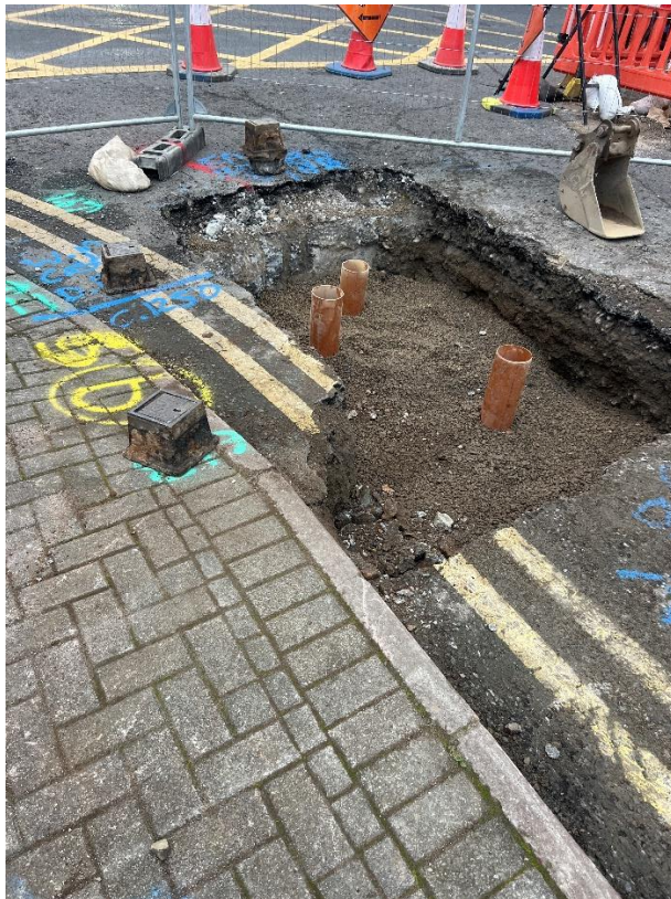
Date: 07 th November 2024 Sluice Valves Kerb Clashes Investigation - Backfilling
