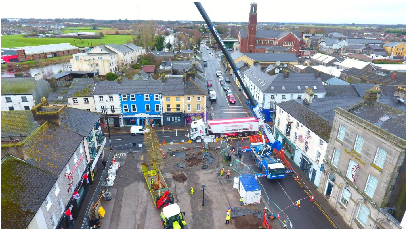
Date: 07 th Feb 2025 Town Tree Installation
