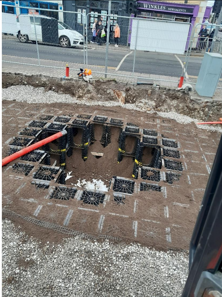
Date: 17 th January 2025 Topsoiling of Tree Pit
