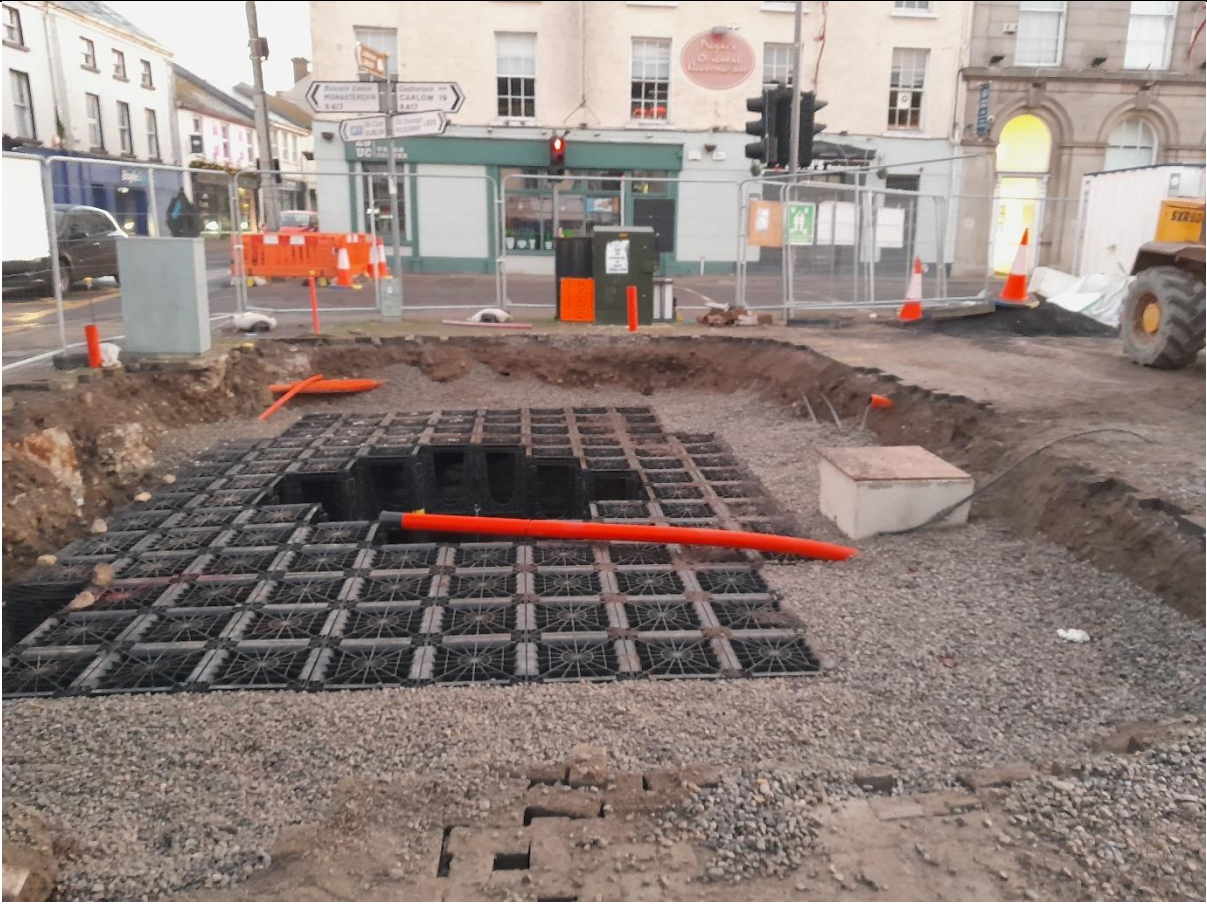
Date: 17 th Jan 2025 Tree Pit Installation ongoing
