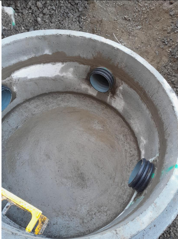
Date: 16 th January 2025 Installation of Manhole S2
