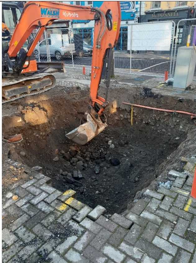
Date: 02-Jan-2025 Excavate Tree Pit
