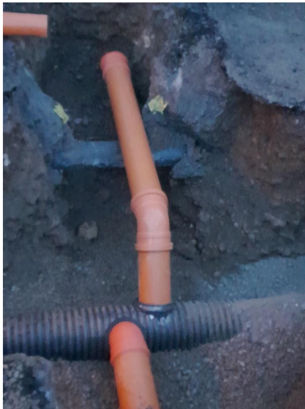
Date: 20 th Jan 2025 Storm Saddled Connections
