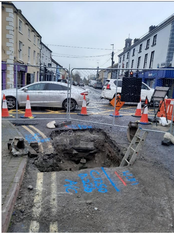
Date: 07 th November 2024 Sluice Valves Kerb Clashes Investigation
