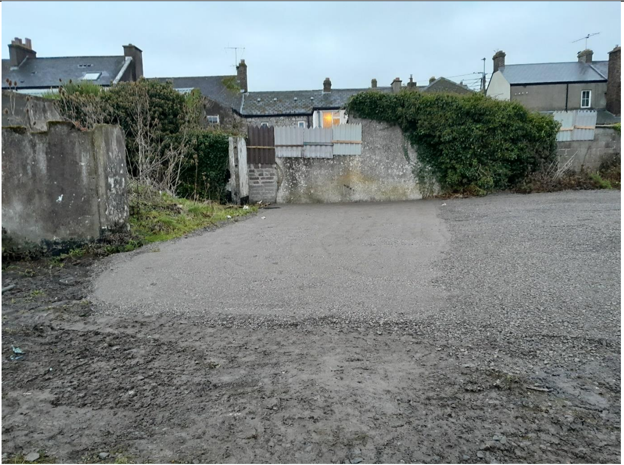
Date: 13 th Jan 2025 Site Compound Set Up
