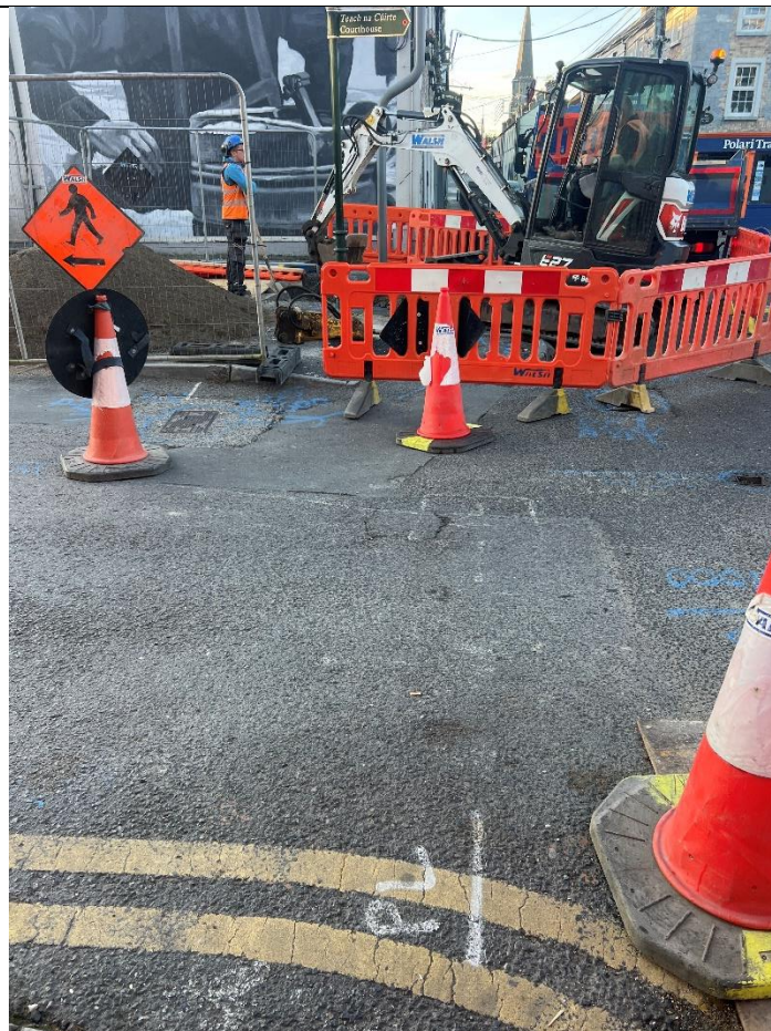
Date: 16 th Sept 2024 Meeting Lane Junction – ESB Duct Installation
