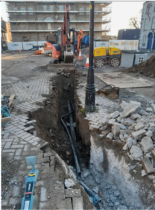
Date: 19th December 2024 Investigate Power Ducting
