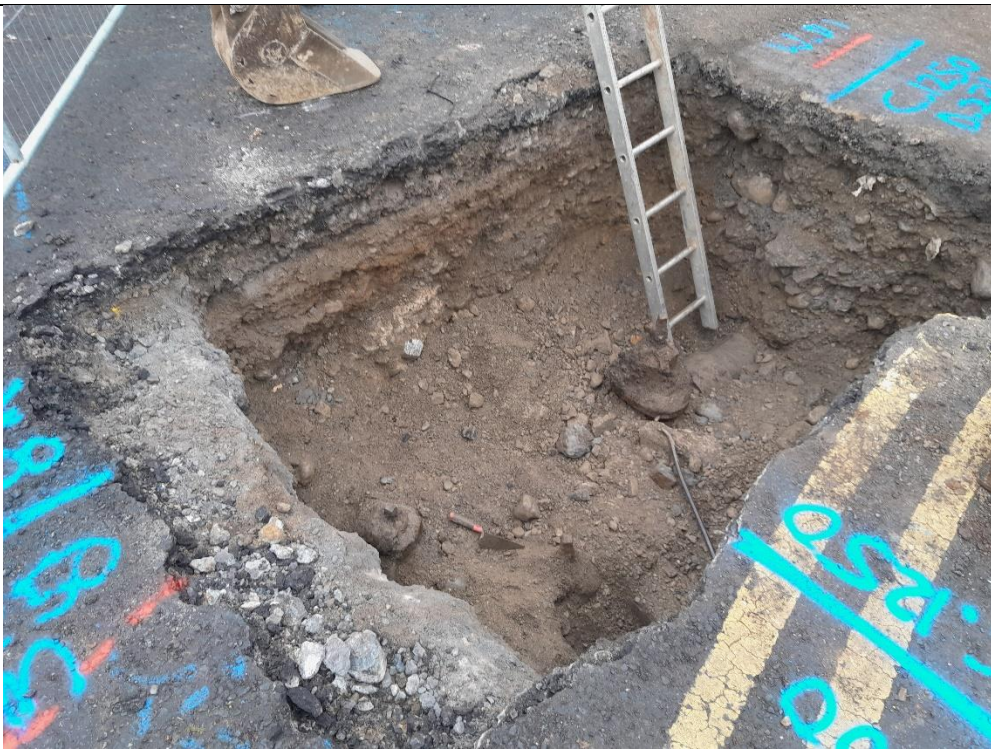
Date: 07 th November 2024 Sluice Valves Kerb Clashes Investigation
