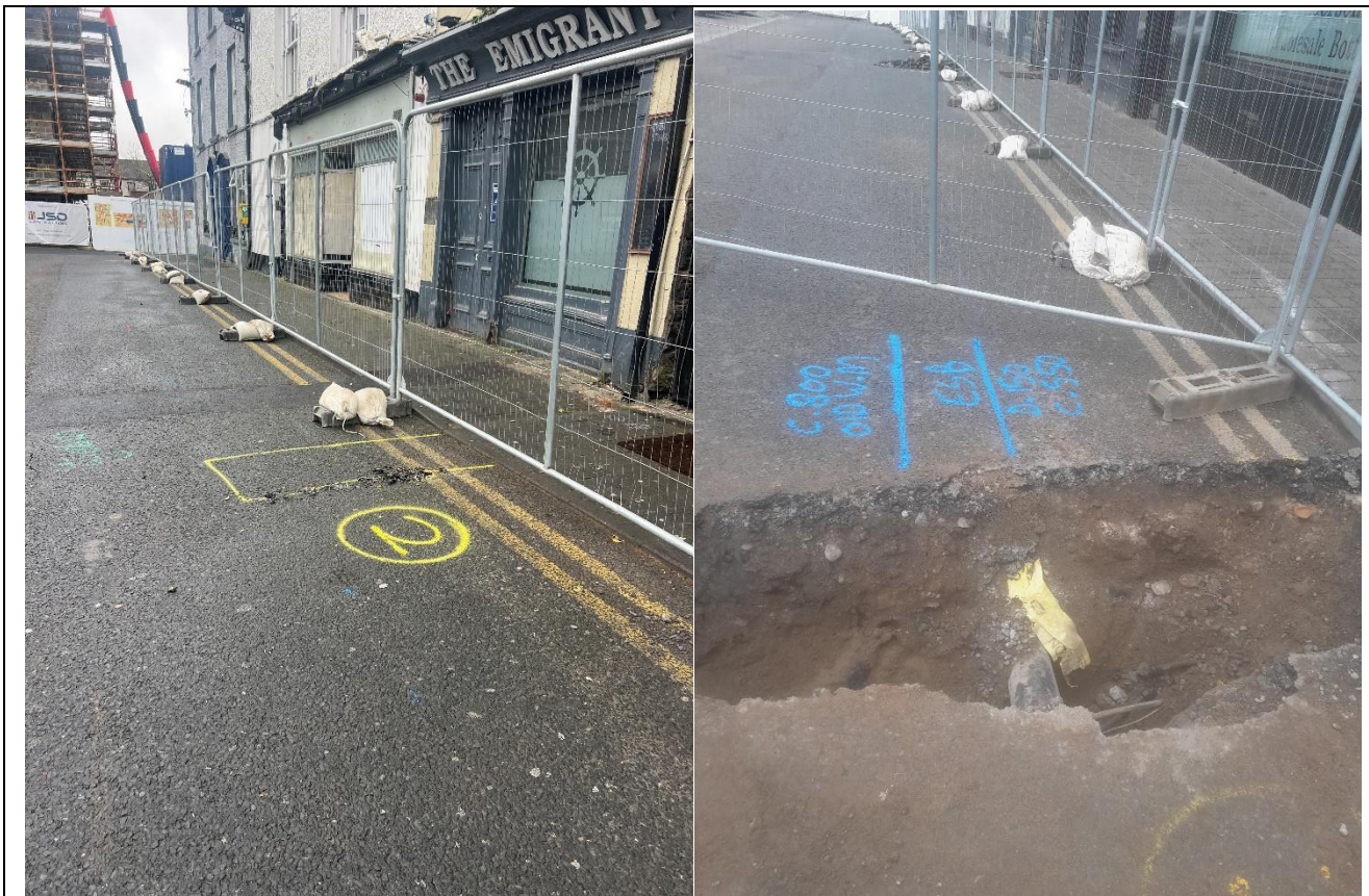
Date: 07 th November 2024 West Side – Watermain Service Connections Investigations
