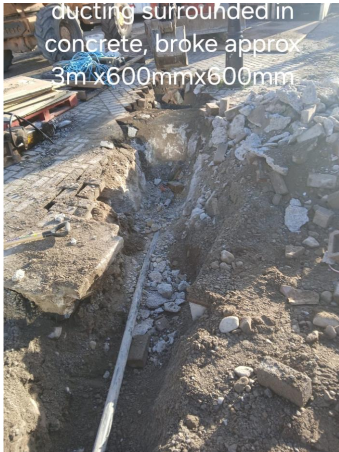
Date: 19 th December 2024 Investigate Power Ducting
