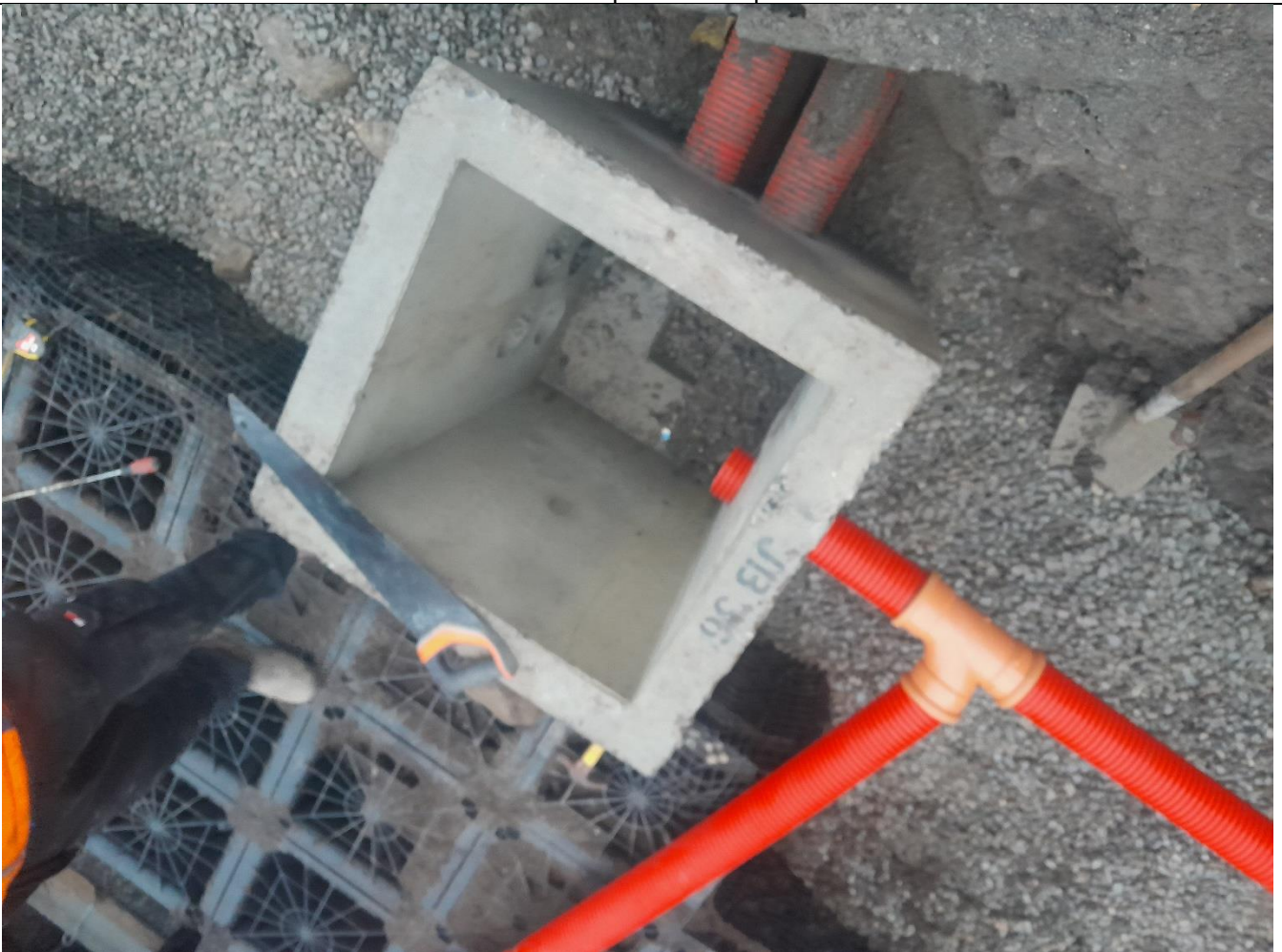
Date: 13 th Jan 2025 Power Ducting and Chamber Installation.
