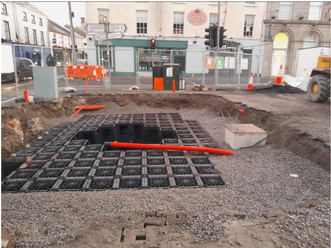
Date: 17 th January 2025 Installation of drainage Stone Around Tree Pit
