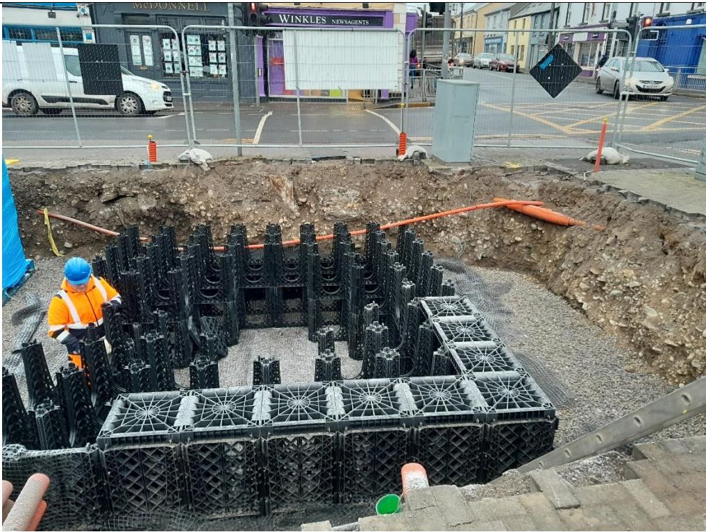
Date: 10 th Jan 2025 Tree Pit Cell Assembly Ongoing
