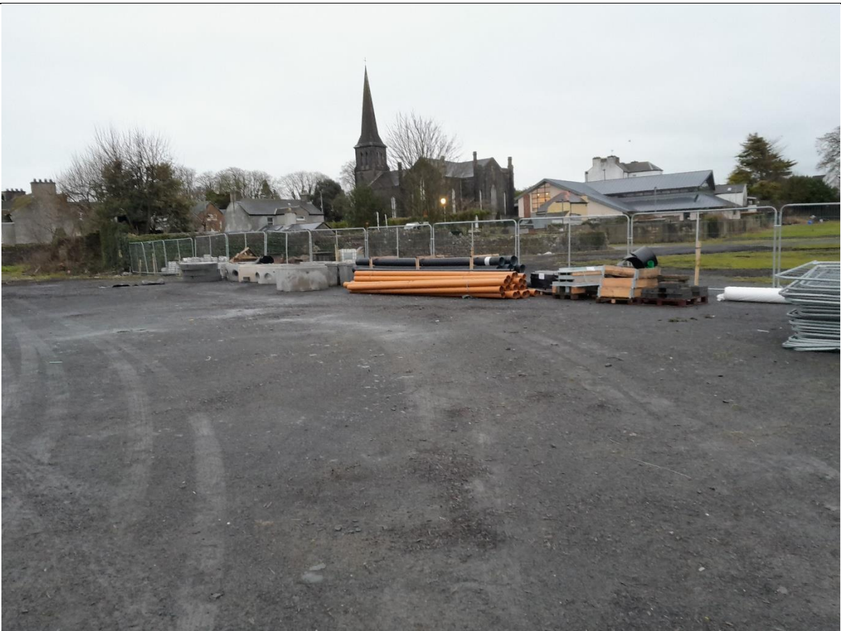
Date: 13 th Jan 2025 Site Compound Set Up
