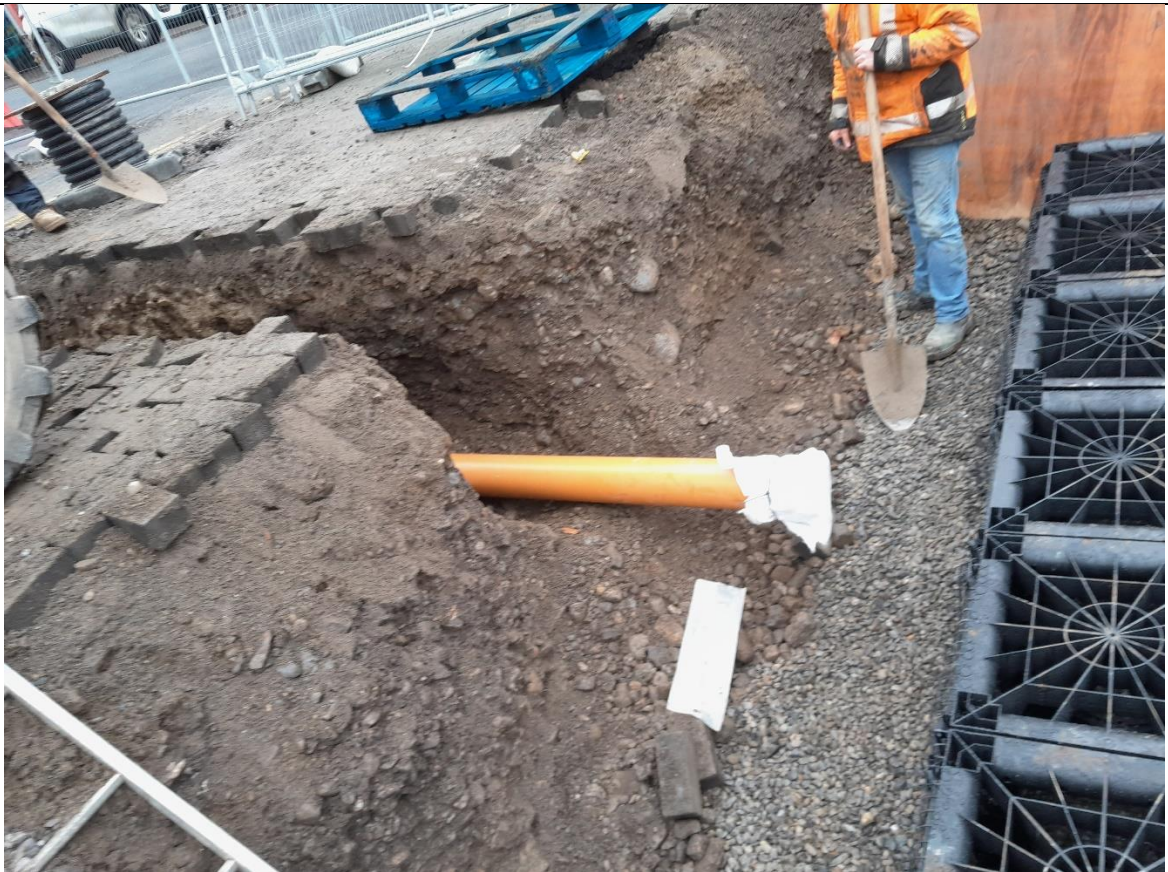
Date: 13 th Jan 2025 Tree Pit Drainage Connection
