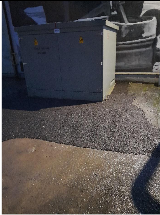
Date: 18 th December 2024 Temporary Reinstatement around ESB Substation
